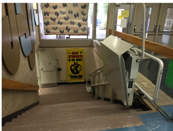
Lift from main school in narrow stair
