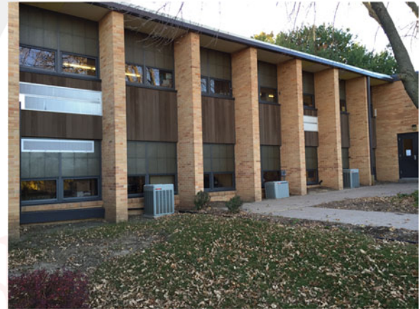
Multiple condensing units at building perimeter are prone to vandalism.
